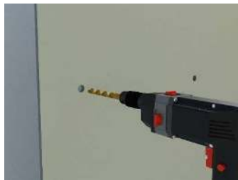
Step 2 Drill holes Use drill bit size 1/2"
