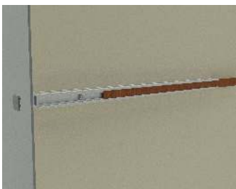
Step 9 Insert provided inlay strip and secure end caps on both sides
