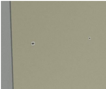
Step 7 Bend until plastic cracks, flush to the wall
